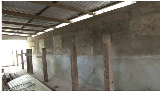
Damaged wall being repaired
